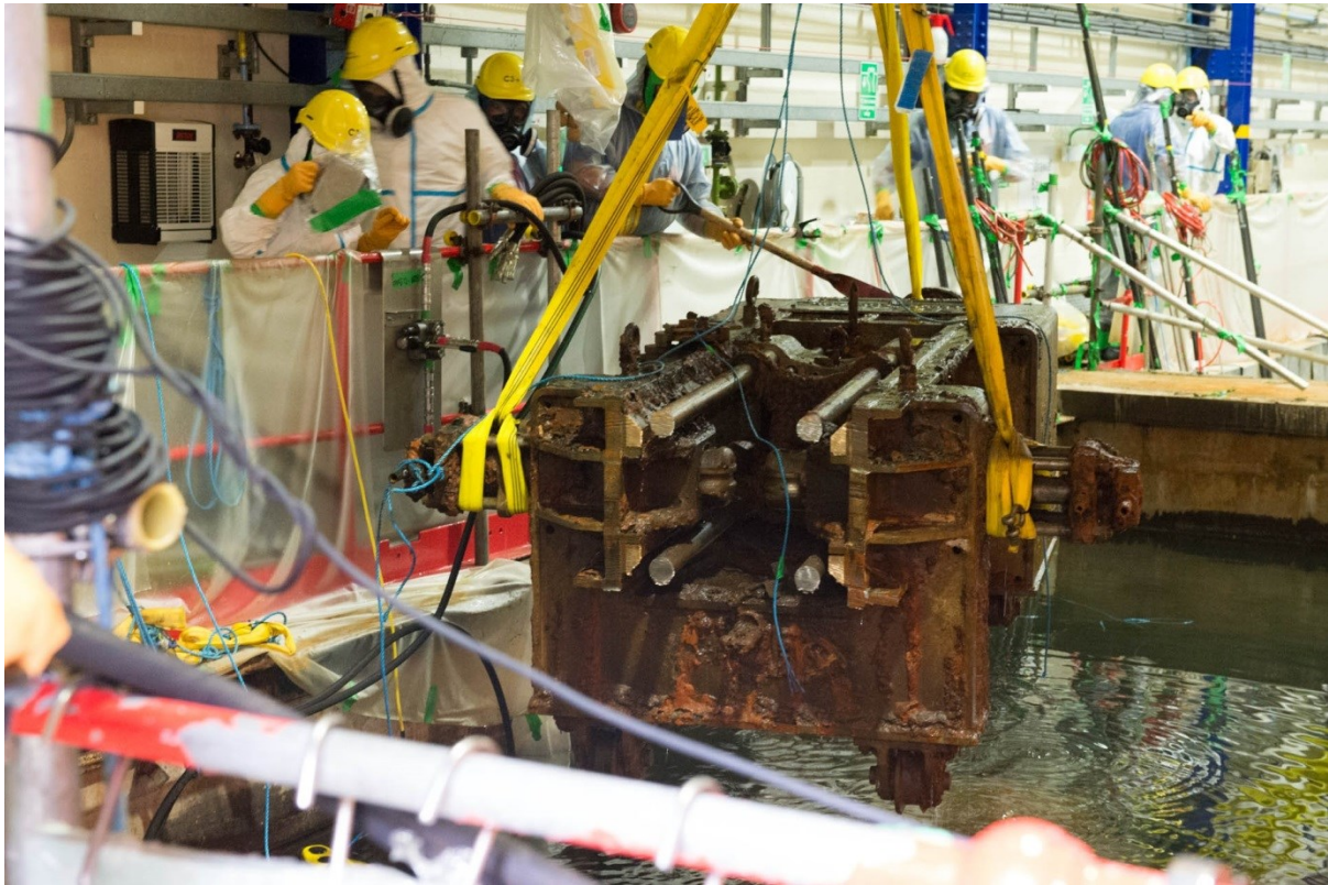
Retrieval of decanner section from legacy pond, Sellafield
