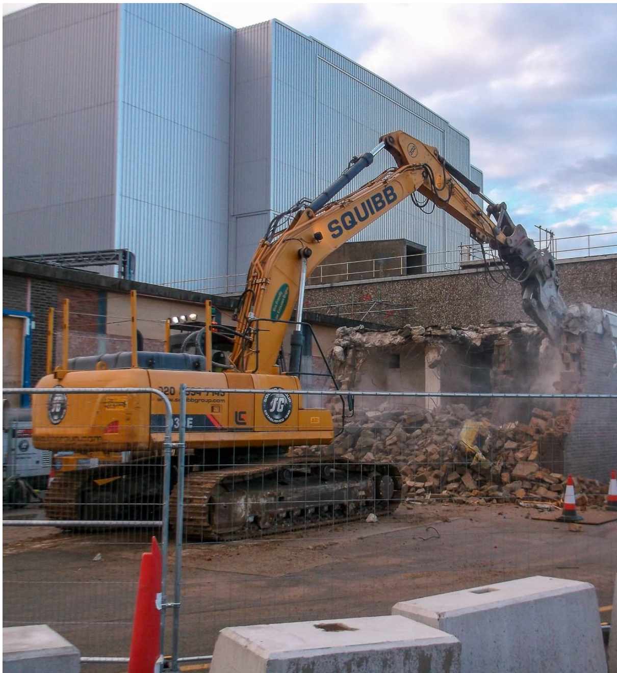
Demolition of former ponds complex at Bradwell Magnox station
