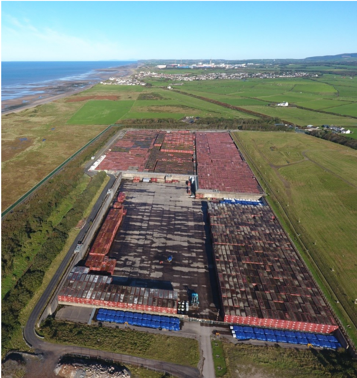
Aerial view of LLW repository
