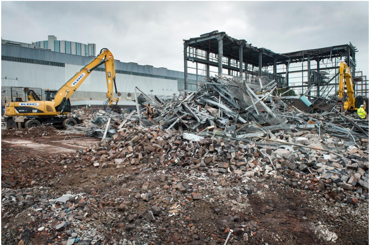
Demolition at Oldbury Magnox station
