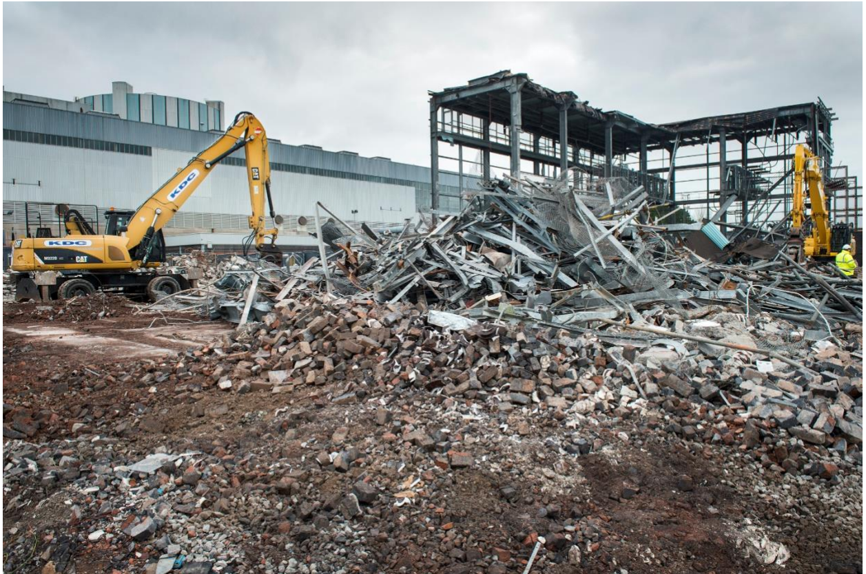
Clearing land at Oldbury
