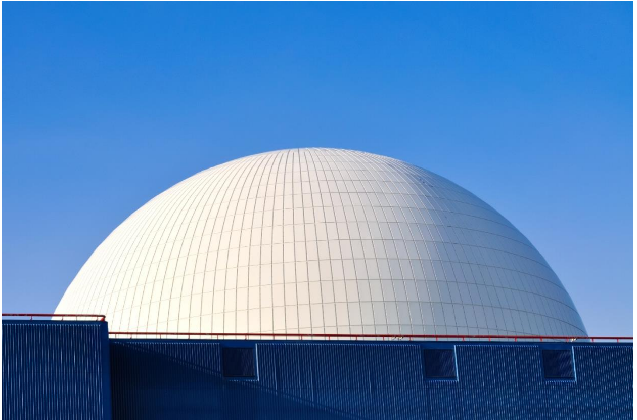
Sizewell B power station
